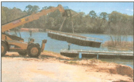
They will be lifted into the water
