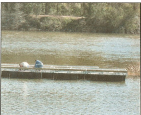
NAMI personnel bolting pieces together
