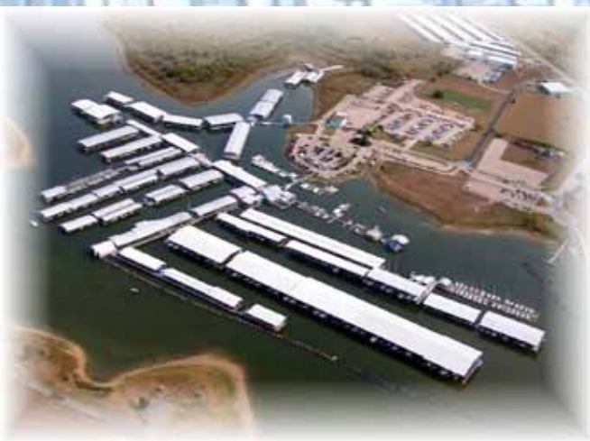
Pier 121 Lake Lewisville, TX
